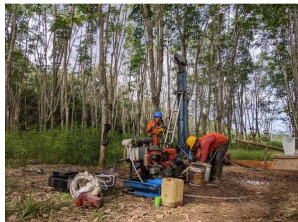
Drilling process at APE site
