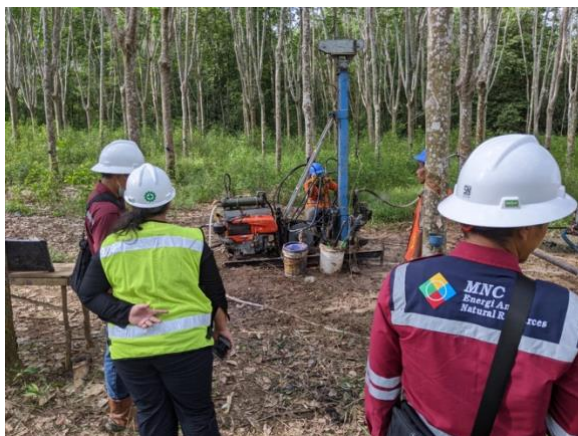
Drilling process at APE (Arthaco Prima Energi) site
